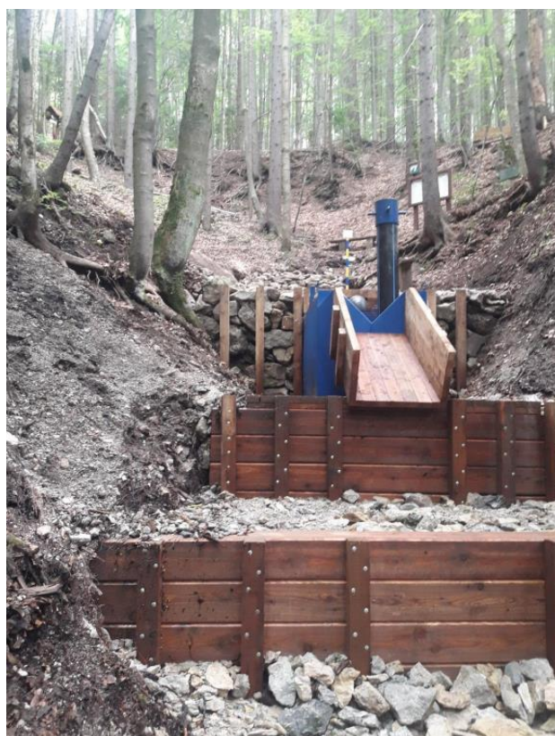
Občasný prameň spring under the Havrania skala Mt. after the reconstruction of gauging object in June 2023. Photo: Ján Gavurník
