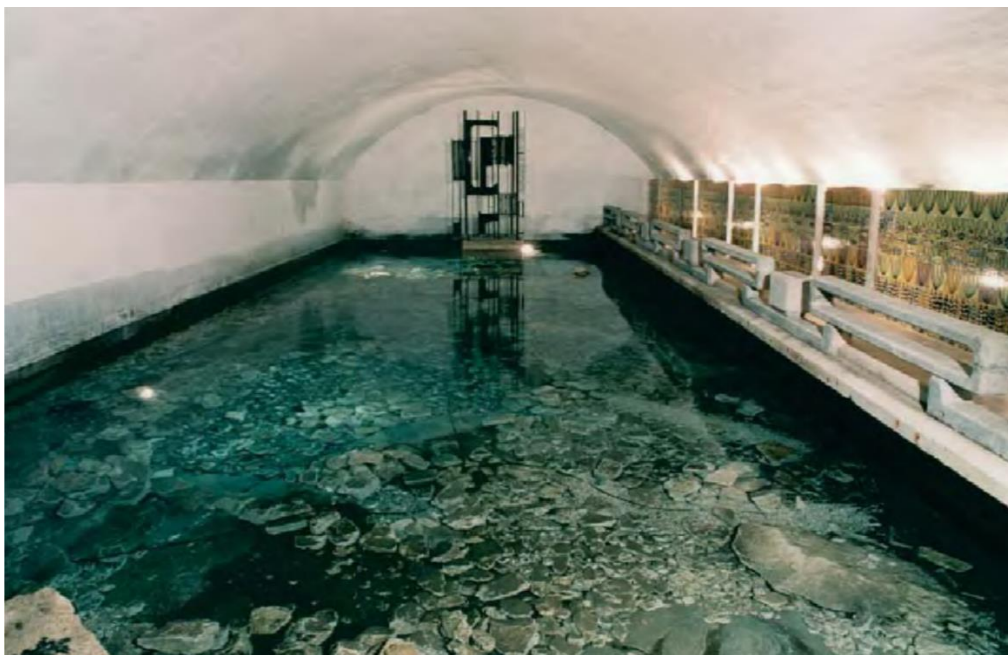
Interior of tapping structure of Peschiera spring (Photo by F. Fiorillo)
