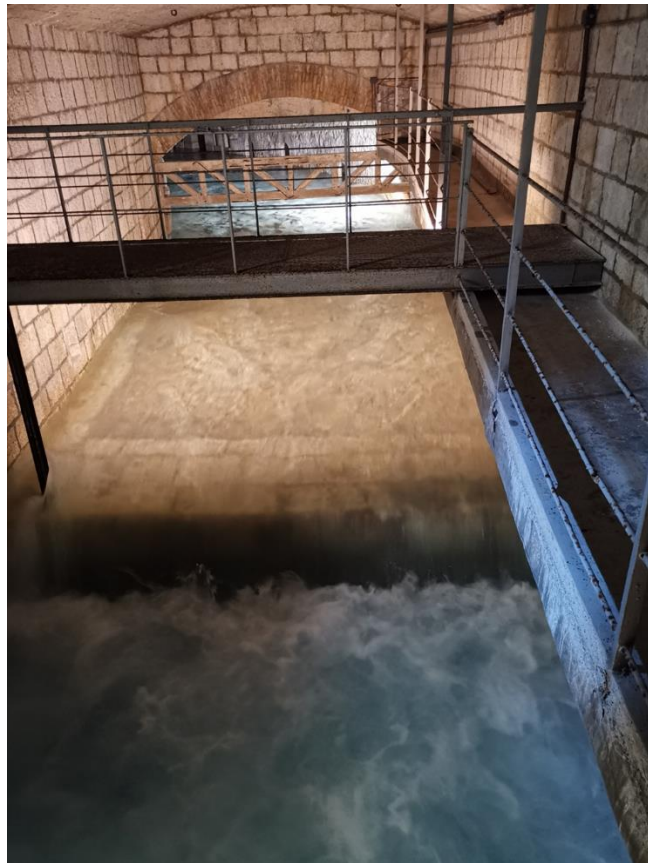
Interior of tapping structure of Sanità spring (Photo by F. Fiorillo)
