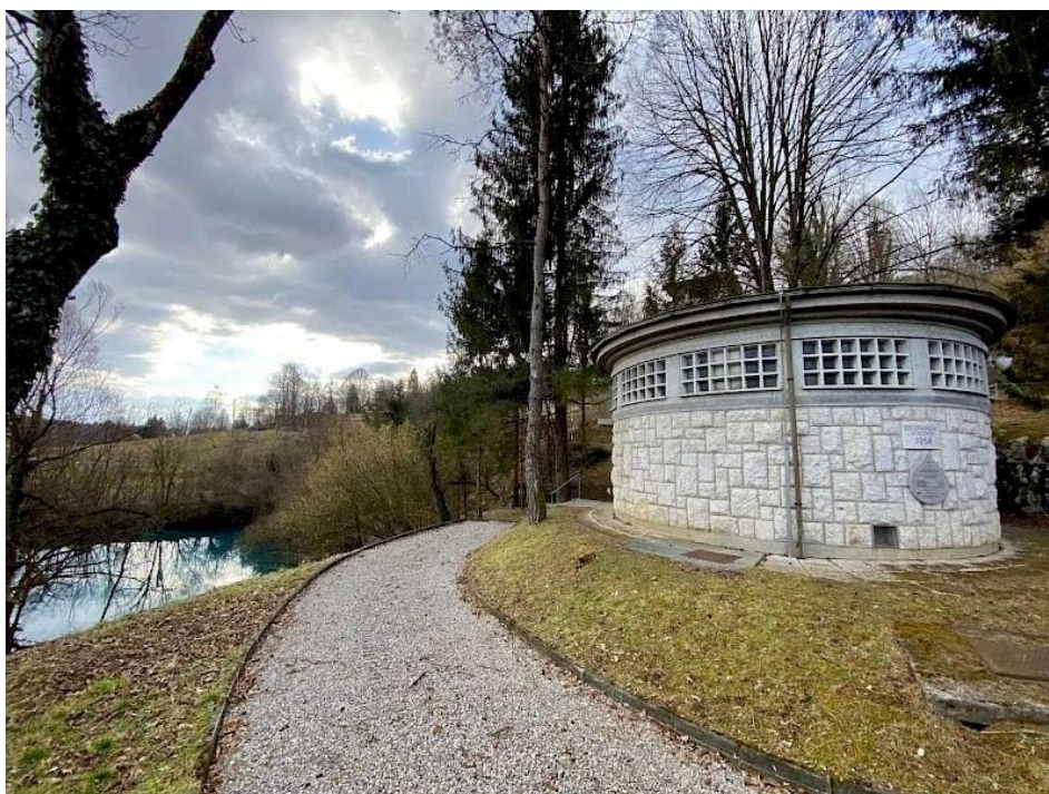
Pumping station at the Dobličica spring ( https://www.radio-odeon.com/novice/crpalisce-v-doblicah/ )
