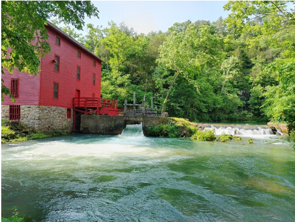
Alley Spring, Missouri, and the mill that are part of the Ozark National Scenic Riverways. Visual estimate of intermediate spring discharge is provided by flow over dam on right side of mill (Photo Z. Stevanović)
