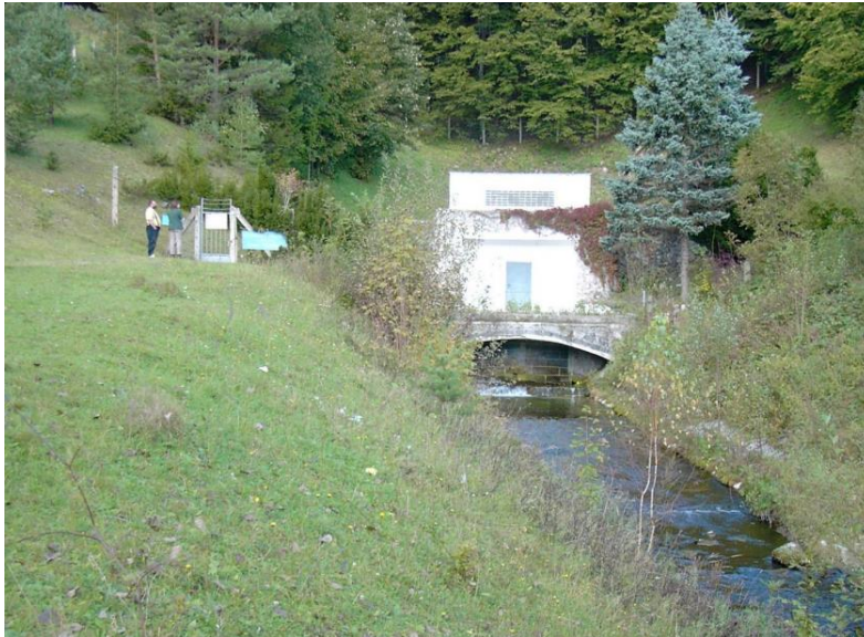
General view of the waterworks intake facility object of the Podhrad spring in Muráň. Photo: Peter Malík.
