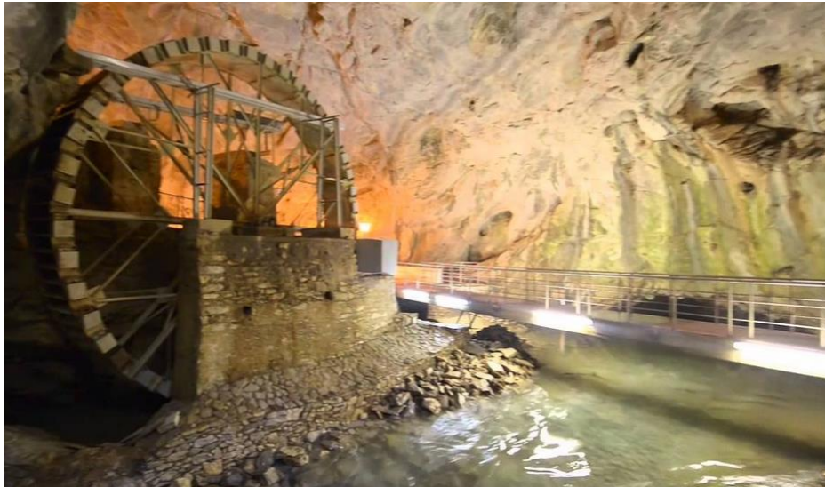
Pumping system in Maaras Cave entrance / Aggitis Spring
