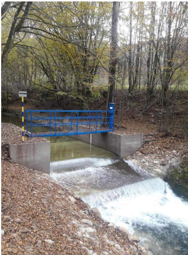
Slovak Hydromet Institute (SHMI) gauging object under the waterworks intake facility object of the Podhrad spring in Muráň at average water stages. Photo: SHMI, taken from www.shmu.sk .
