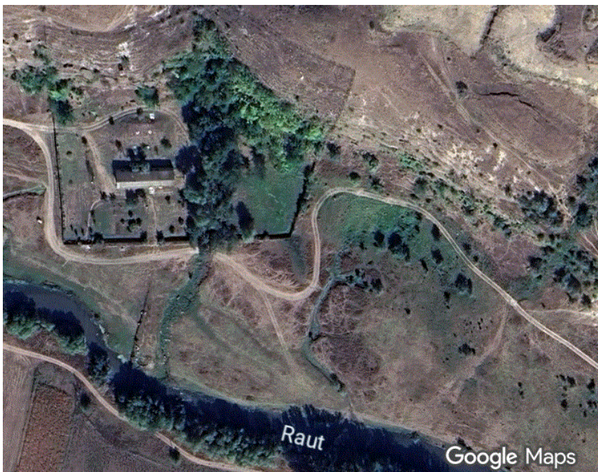
Jeloboc water pumping station near Raut riverbank (Google Maps)
