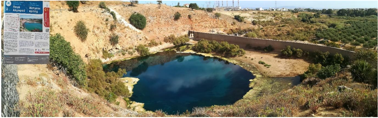
Almyros dam and informative panel (photo by Z. Stevanović)
