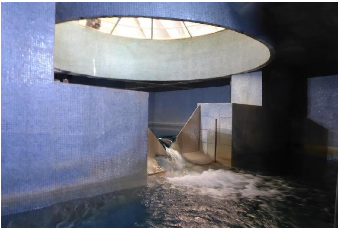
Thomson's culvert gauge in the Vrchovište spring waterworks intake facility (SHMÚ object no. 1095). Photo: Peter Malík.
