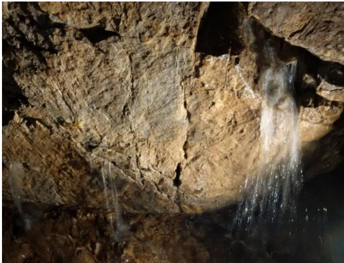
Groundwater discharging from fissures of scratched carbonates in the waterworks facility of the Bobrovec (Bobrovecká dolina) spring. Photo: Peter Malík.
