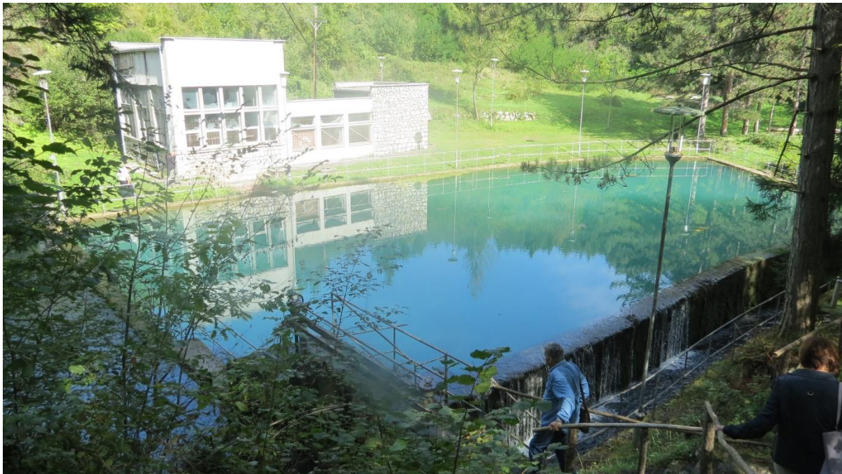
Intake and overflow of the Vrelo Raške (Photo Z. Stevanović)
