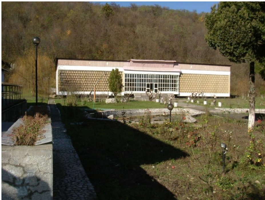
Main building of Izvarna intake structure (photo by Carlan Constantin)
