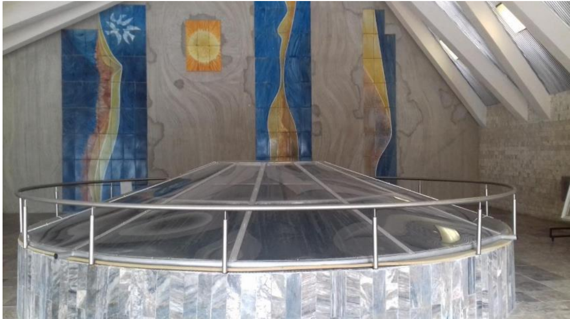
Interior of the hall of the Vrchovište spring waterworks intake facility in Slatinka nad Bebravou. Photo: Peter Malík.
