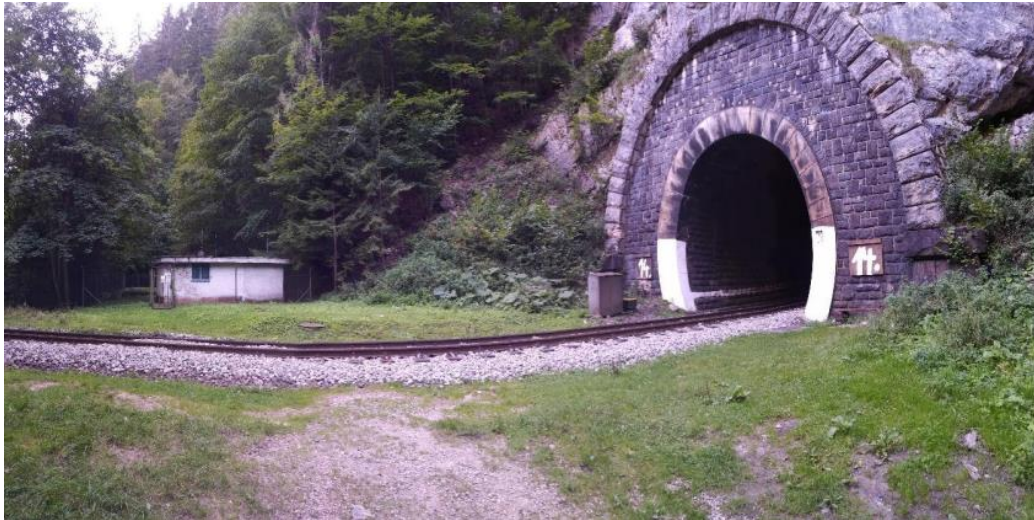
Eastern portal of the Čremošný tunnel, in the background the Harmanecký Veľký tunnel water intake. Photo: Peter Malík.
