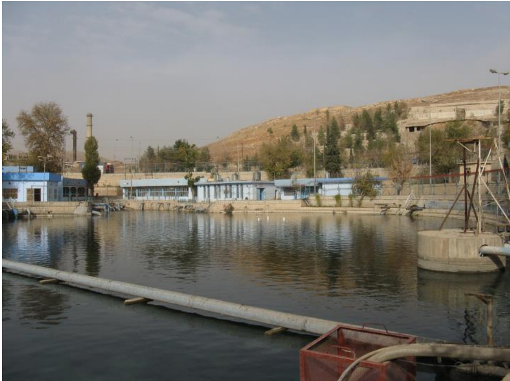
Pumping station of the ascending spring Sarchinar (photo: Z. Stevanović)
