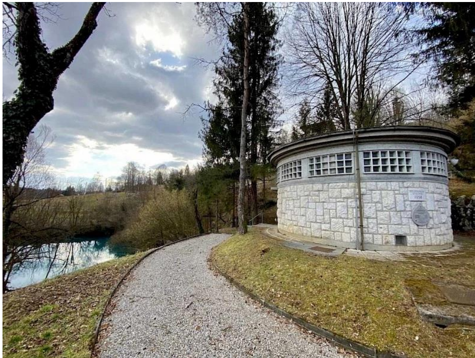
Pumping station at the Dobličica spring ( https://www.radio-odeon.com/novice/crpalisce-v-doblicah/ )
