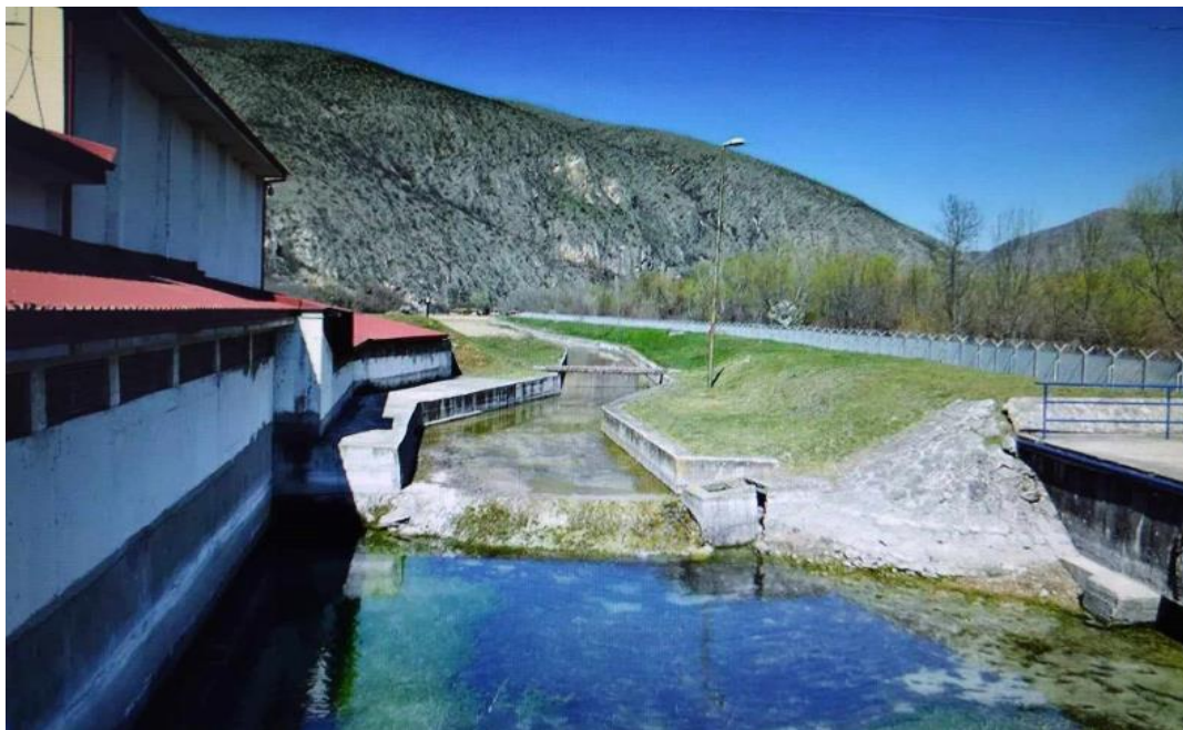
The intake Rashche 2 and a channel for diverting overflow into the nearby Vardar River
