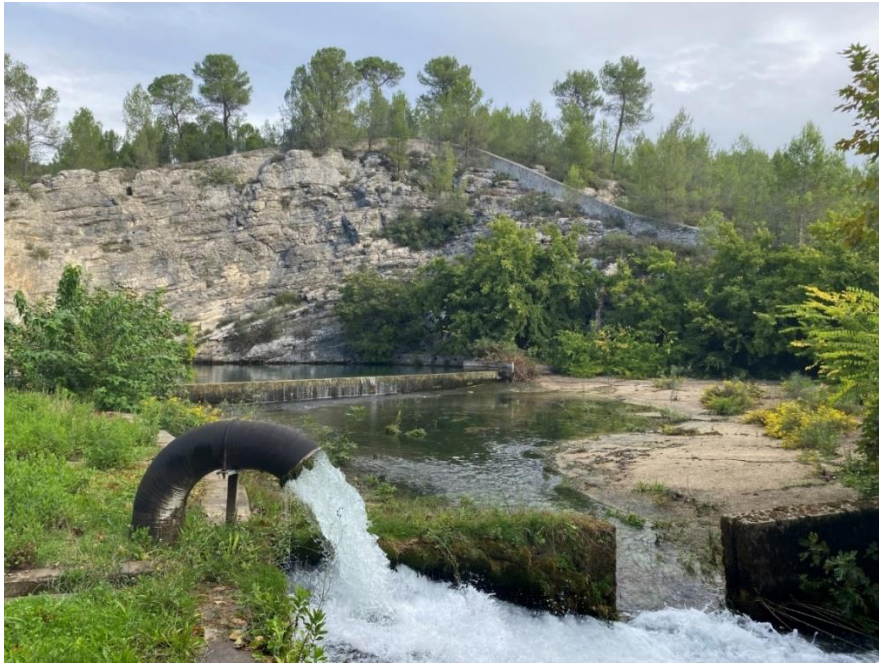
Ecological flow diverted towards the Lez river when the natural discharge becomes insufficient (photo H. Jourde).
