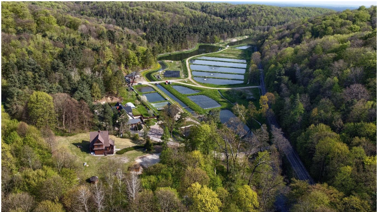
Photo of the contemporary Trout House (Photo by P. Kokoszka)
