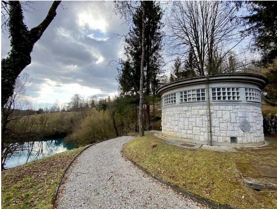
Pumping station at the Dobličica spring ( https://www.radio-odeon.com/novice/crpalisce-v-doblicah/ )
