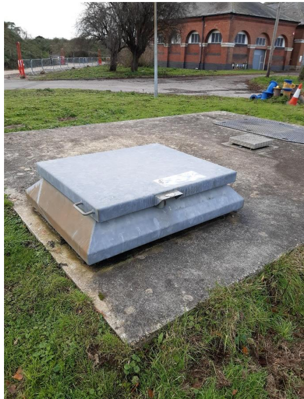
Spring upwelling hatch at the Public Water supply site (Photo copyright Portsmouth Water)
