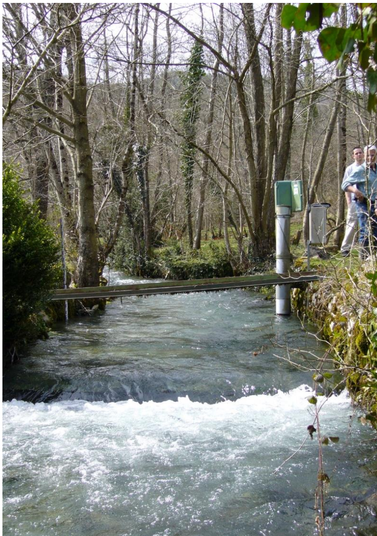
The main hydrometric station, downstream Las Hountas, controlling the total flow from the main spring and the overflow springs (photo D. Labat).
