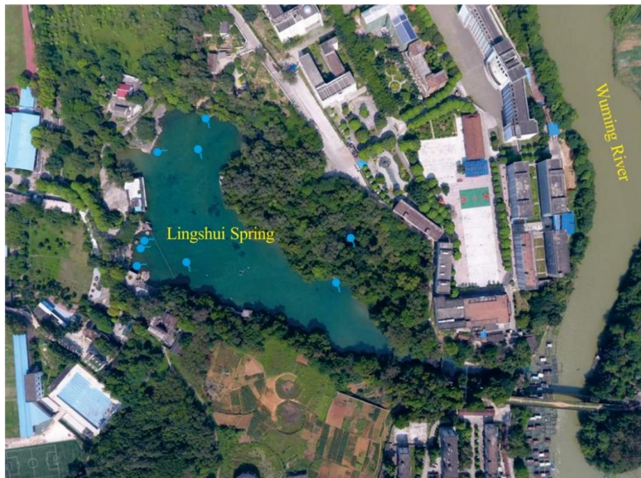
Lingshui spring in SW China. Detailed view, depicting the positions of the nine spring outlets and the Wuming River.
