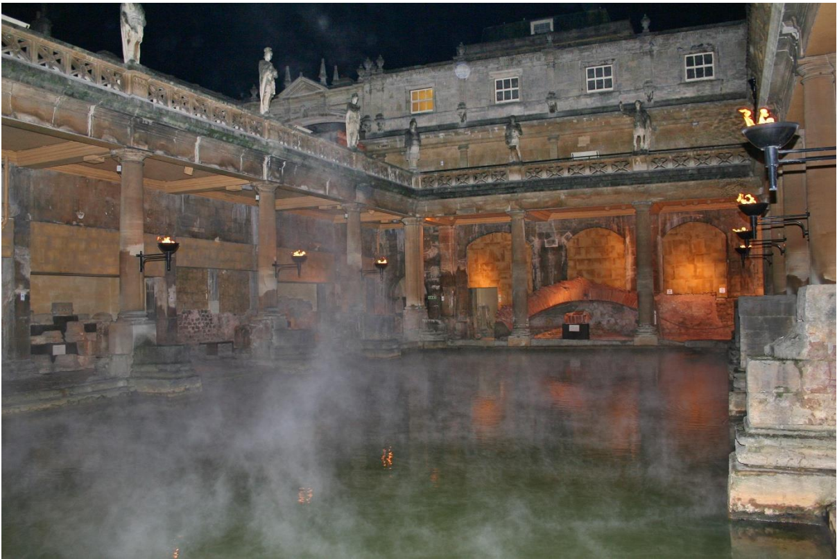
The old thermal baths fed by hot springs (photo copyright Alan Gray)
