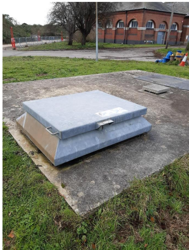
Spring upwelling hatch at the Public Water supply site (Photo copyright Portsmouth Water)
