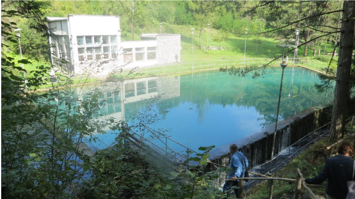
Intake and overflow of the Vrelo Raške (Photo Z. Stevanović)
