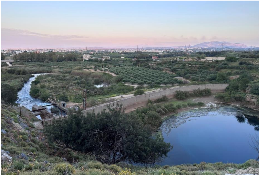
Overview of Almyros dam, Crete Island, Greece (Photo by H. Bouloukakis)
