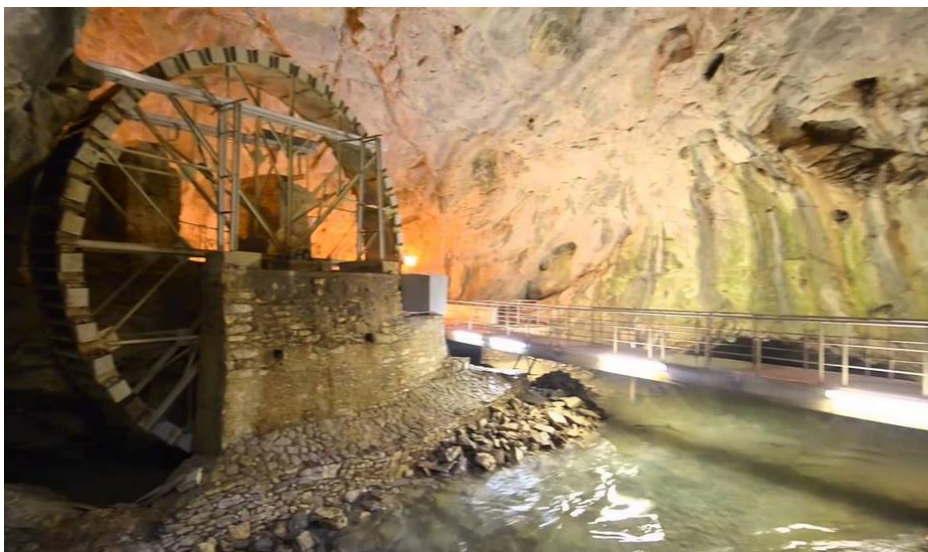
Pumping system in Maaras Cave entrance / Aggitis Spring (courtesy of K. Voudouris)
