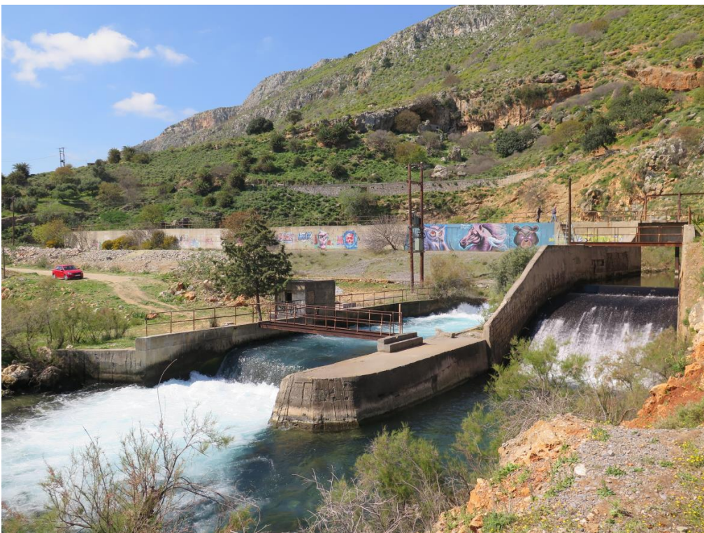
Almyros dam, Crete Island, Greece (provided by V. Perleros)
