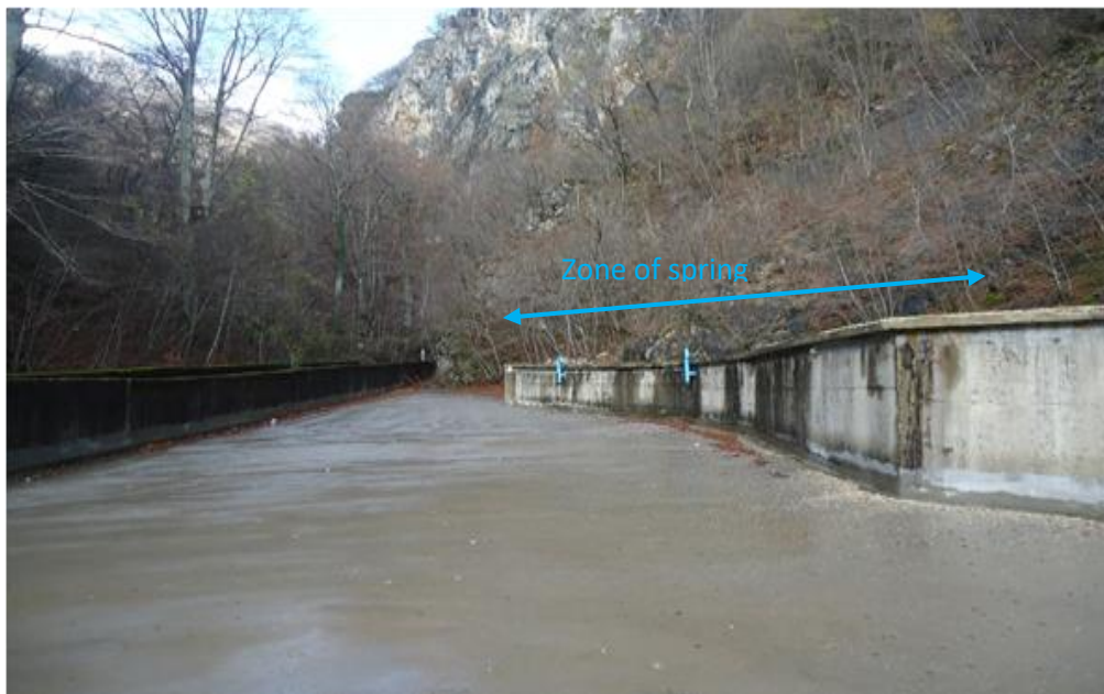
Reinforced concrete slab above the intake structure/collection channels and the spring of Studenchica
