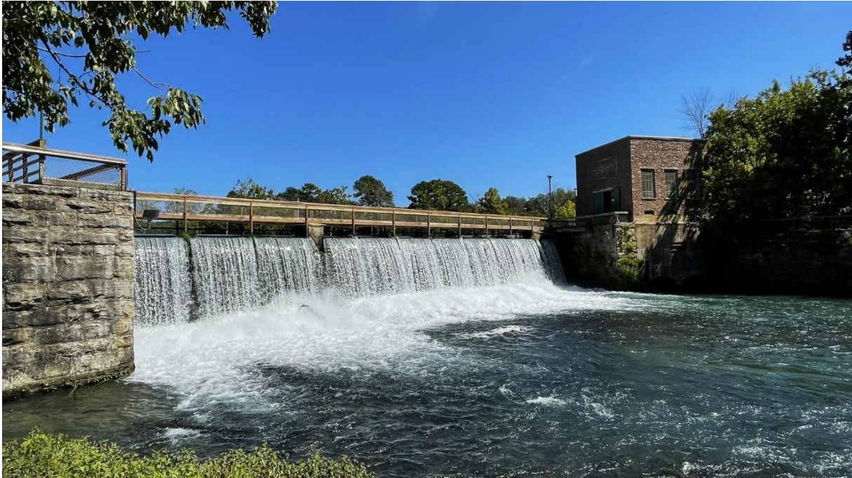
Hydroelectric dam at the distal end of the spring run of Mammoth Spring, Arkansas, where the spring water flows over the dam and creates the headwaters of the Spring River. The hydroelectric aspects of the structure are no longer operational (Photo by Neven Kresic)
