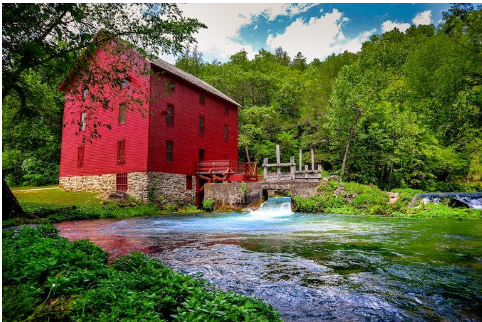
Image of Alley Spring, Missouri, and the mill that are part of the Ozark National Scenic Riverways. Visual estimate of intermediate spring discharge is provided by flow over dam on right side of mill (Photo credit: Lucas Bremer. https://www.theoutbound.com/missouri/photography/explore-alley-spring-and-mill-within-the-ozark-national-scenic-riverways/photos#photo-308145 )
