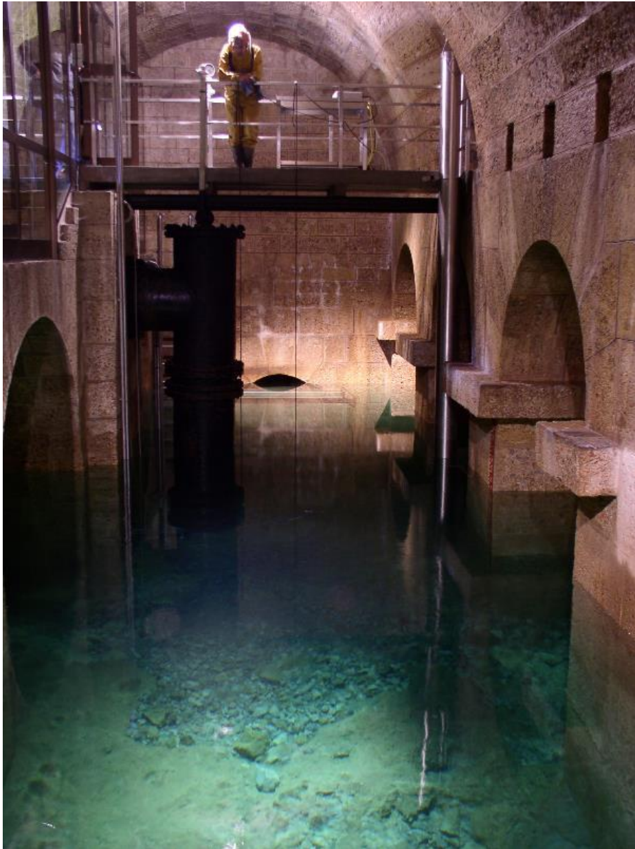
Interior the spring capture building of Kaiserbrunnen (Photo: L. Plan)
