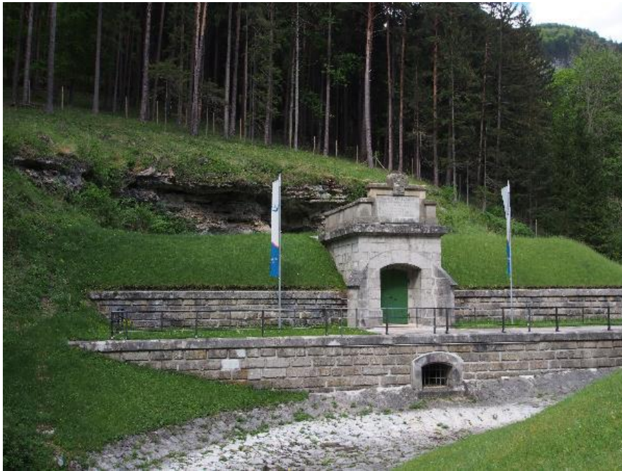
Spring capture building at Kaiserbrunn (Photo: L. Plan)
