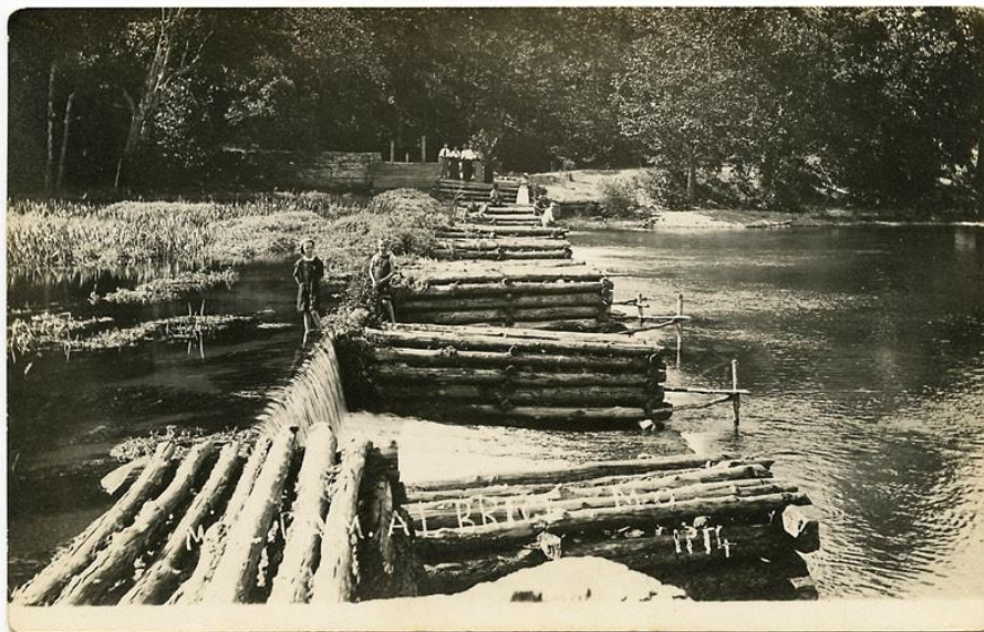
Historic image from a 1914 post card shows a crude wood structure seen here blocking the spring run from Brice Springs – now called Bennett Spring. Bennett Spring is now a Missouri state park. Photo credit: http://www.dammingtheosage.com/brice-spring-now-bennett-spring-state-park-on-the-niangua-river/
